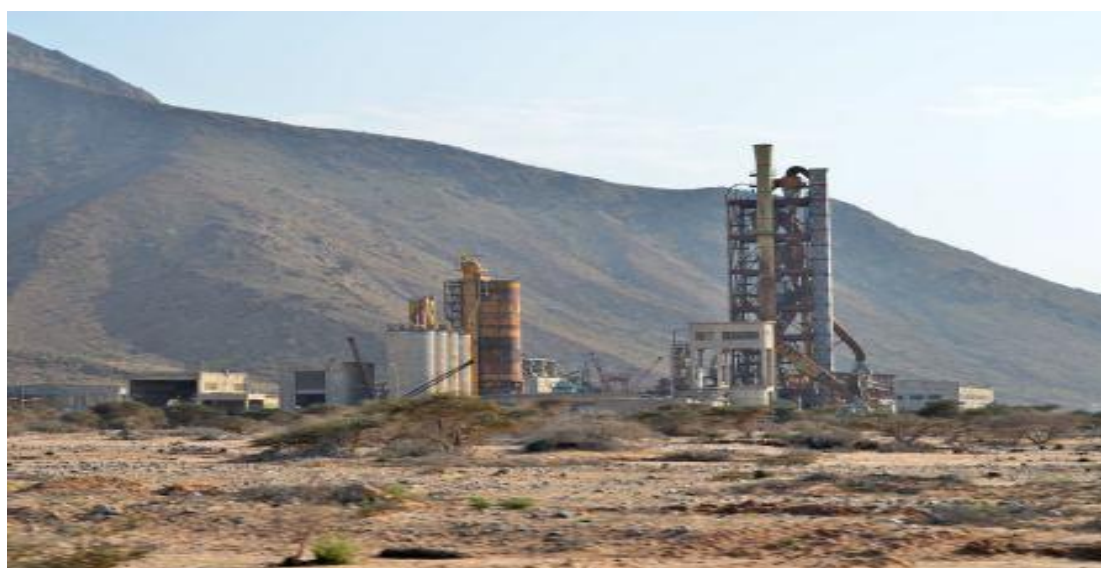
Figure 21: A photo of the derelict cement factory in Berbera
